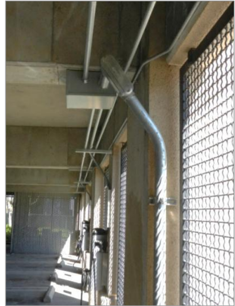
Ceiling-mounted conduit located near wall
