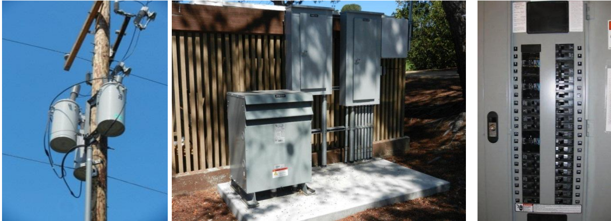
From left to right: (1) pole-mounted transformers; (2) surface-mounted transformer and electrical panels; (3) circuit breakers in electrical panel
