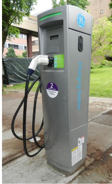
Level 2 EV supply equipment
