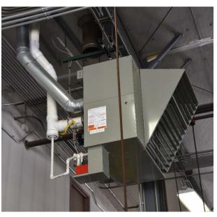
Sealed-combustion or separated-combustion unit heaters can be used in the vehicle space. Users must confirm that the unit is fully sealed and that no surfaces exceed 750°F.
