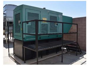
Required for gas detection systems (2018 IFC Section 916.5). It is best practice to provide a standby generator to power the gas detection system, fans, overhead doors, lights and other safety-related equipment.
