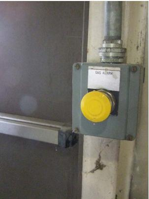
Provide manual gas detection activation buttons at man doors to allow staff to manually put the system in Level 2 response.
