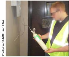
Equip the system for "Floor Level Calibration" to avoid the need and cost of using a lift to calibrate detectors (see tubing on detector that is routed to floor level).
