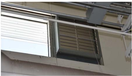
Wall-mount type fan mounted in a clerestory which forms a high point and natural collection point for lighter-than-air gases.
