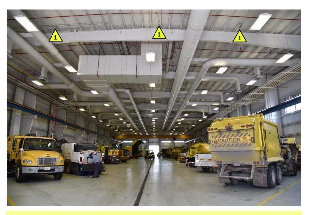
1. Catalytic type combustible gas point detectors located in 3 rows above bays and at peak of maintenance shop areas.
