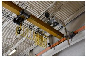
Using a contactor to remove power from the bridge crane eliminates a potential ignition hazard (open buss bars). The contactor is controlled by the gas detection system.
