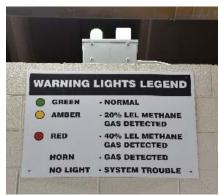
Provide highly visible status lights inside the garage and outside above overhead doors.
