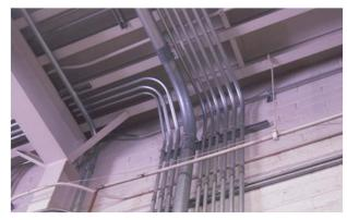
The many conduits above would be very expensive to relocate or upgrade and pose very little sparking risk. Most retrofit garage upgrades use the 1 cfm/ft<sup>2</sup> exemption from the Class I, Division 2 requirement.
