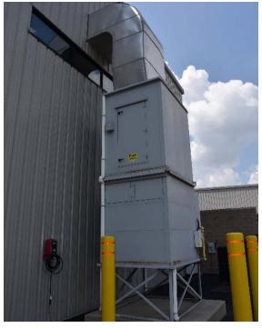
Direct-fired MAUs installed outside of the vehicle space provide a safe, lowcost, high-efficiency heat source. Note that the fan must start and "prove" airflow prior to firing the burner.
