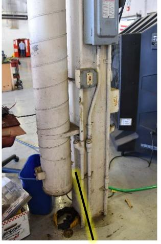
Floor height continuous exhaust—ventilation for LNG vapor as well as conventional liquid fuels.
