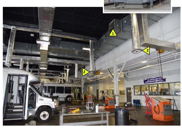
Best Practice Baseline (Continuous) Ventilation for Flat Roof with Precast T-Beams
