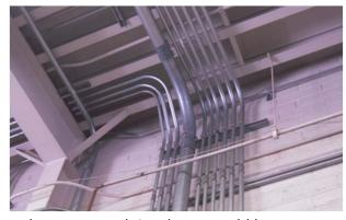
The many conduits above would be very expensive to relocate or upgrade and pose very little sparking risk. Most retrofit garage upgrades use the 4 ACH exemption from the Class I, Division 2 requirement.
