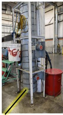
Floor-height continuous exhaust—ventilation for LNG vapor as well as conventional liquid fuels.
