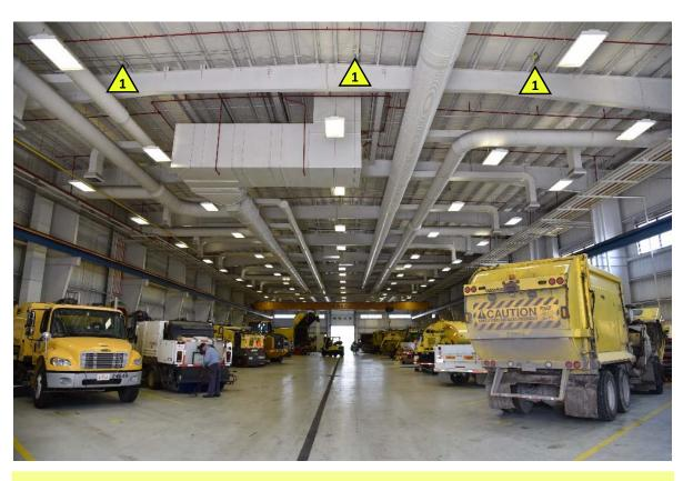
1. IR type combustible gas point detectors located in 3 rows above bays and at peak of maintenance shop areas.
