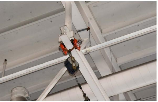
Rail above several bays to provide safe access for cylinder inspections on rooftop-mounted cylinders (refuse trucks).
