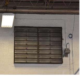
Actuated damper opens when wall-mounted supplemental exhaust fans are operating.
