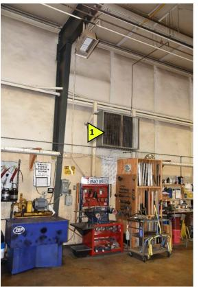
1. A row of 5 evaporative ("swamp") coolers on the wall opposite the overhead doors provide constant floor-level ventilation when the overhead doors are open.
