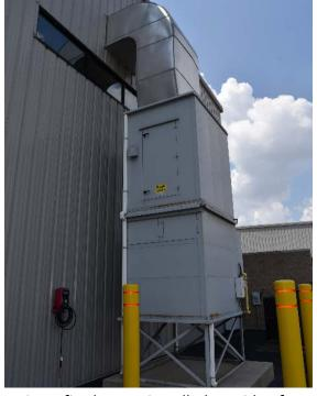
Direct-fired MAUs installed outside of the vehicle space provide a safe, lowcost, high-efficiency heat source. Note that the fan must start and "prove" airflow prior to firing the burner.
