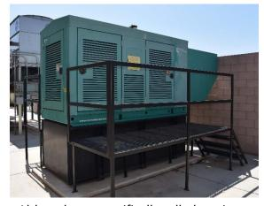
Although not specifically called out in codes, it is best practice to provide a standby generator to power the gas detection system, fans, overhead doors, lights and other safety-related equipment.
