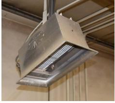
16 non-explosion proof rated catalytic gas heaters provide supplemental heat.
