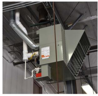
Direct-fired unit heaters can be used in the vehicle space, although sealed-combustion units provide additional safety and improved indoor air quality.
