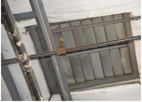
Ceiling-mounted supplemental exhaust fans—manually operated.
